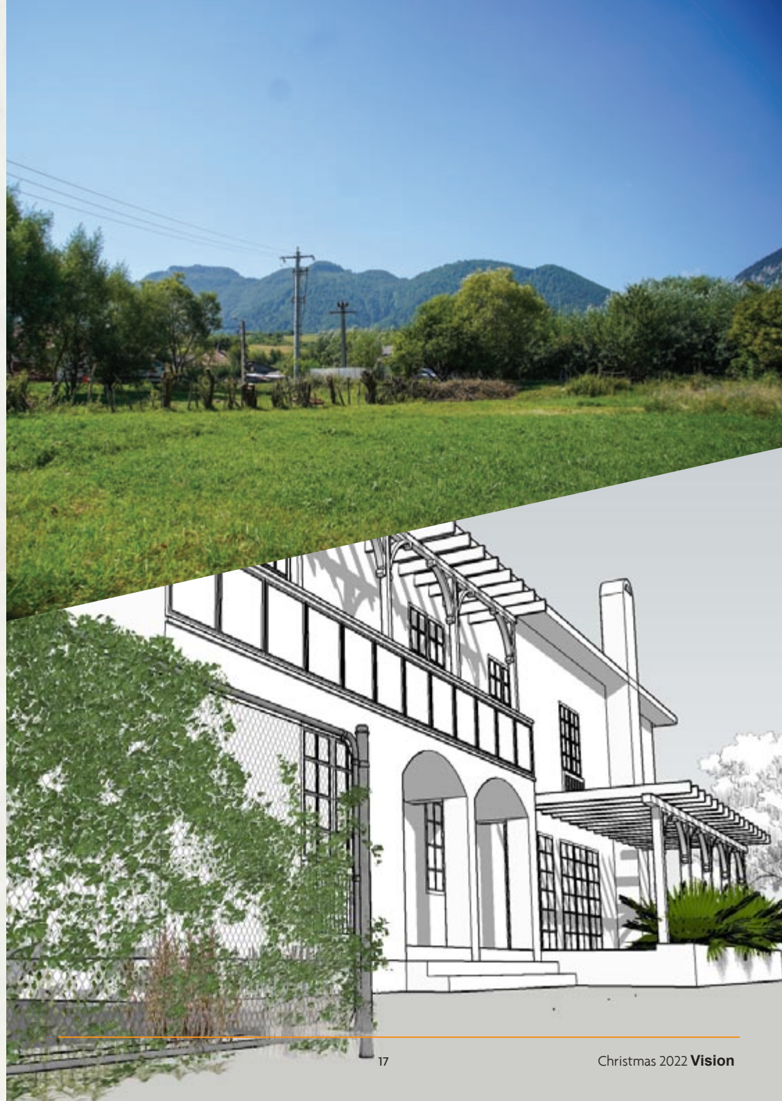
Above opposite: the beautiful location in Zarnesti for Pineview, and below and top visualisations of the building.
